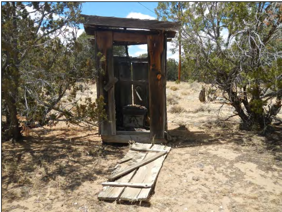
Figure 35: LA 179153 Feature 5 Facing East (top) and Facing Northwest (bottom).
