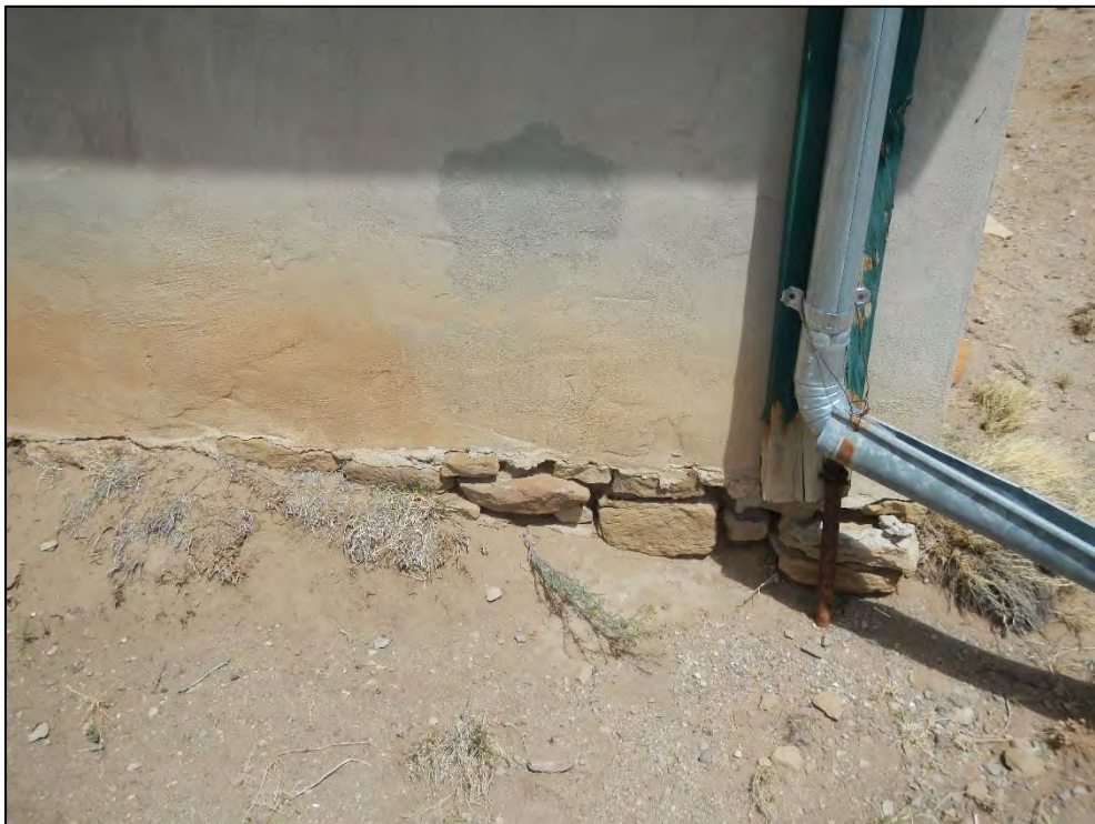
Figure 30: LA 179153 Feature 1 Facing East (top) and Close-up of Foundation (bottom).
