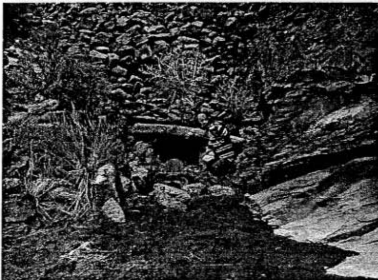
Figure 10: View of the Canyon side outlet at the remains of the Dam. The gate valve works are the only remaining vestiges of the Dam works and are not functional.
