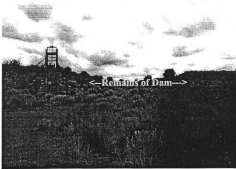
Figure 11: View shows the remains of the Dam and gate valve works from as seen from the Lake. The Dam has been functionally destroyed and would have to be completely rebuilt in order to impound water again.
